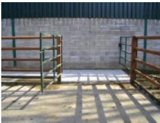
Figure 2: Collecting pens set at 90° to the exit lane may appear as a dead end
