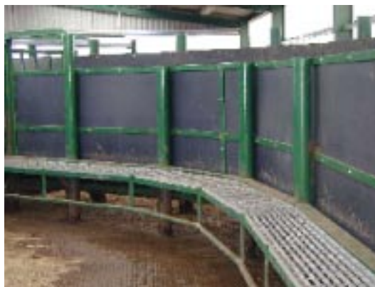
Figure 6: Raised catwalks are necessary with high sided sheeted races
