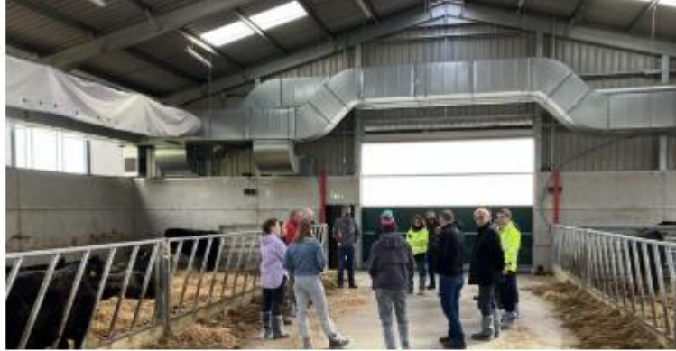
Tour delegates viewing shed internal air conditioning ducting by No Pollution and Galebreaker's ventilation tubes and membrane system.
