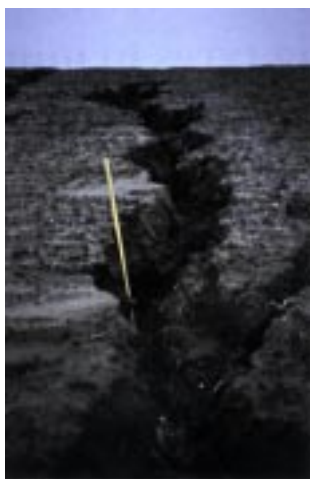
Figure 1 Soil erosion associated with compaction
