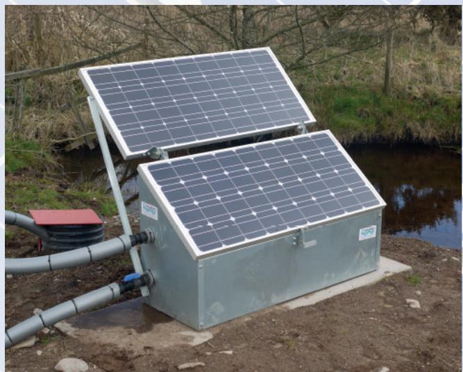
Figure 6: Packaged solar pump unit.
