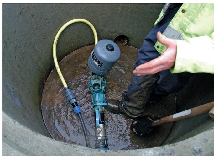
Figure 11. Ram pump within pumping chamber.
