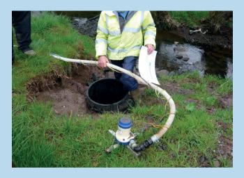
Figure 7: Open abstraction sump chamber for installation of submersible pump.
