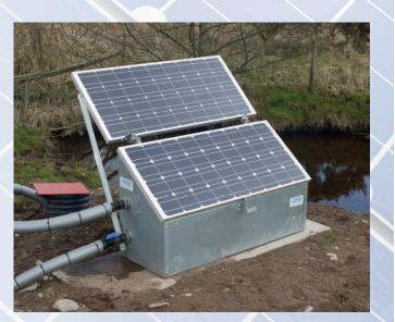
Figure 6: Packaged solar pump unit.
