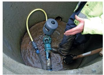
Figure 11. Ram pump within pumping chamber.
