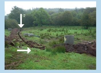
Figure 12: During installation. Note the site for the intermediate break chamber (1) and location of pump and discharge to watercourse (2). Abstraction point is 130m behind photographer.
